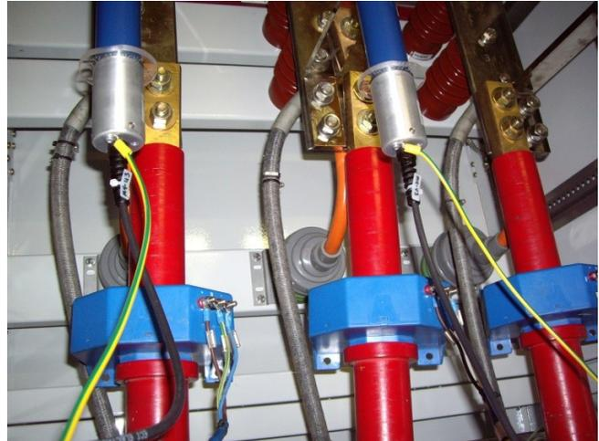
Fig. 2 Installation of the 80 pF capacitive sensors on the motor terminals.
