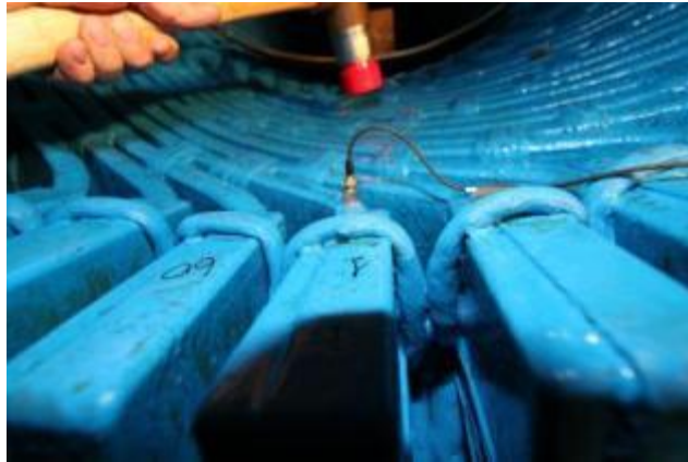
Figure 3. Impact Test Setup with Force Hammer and Accelerometer
