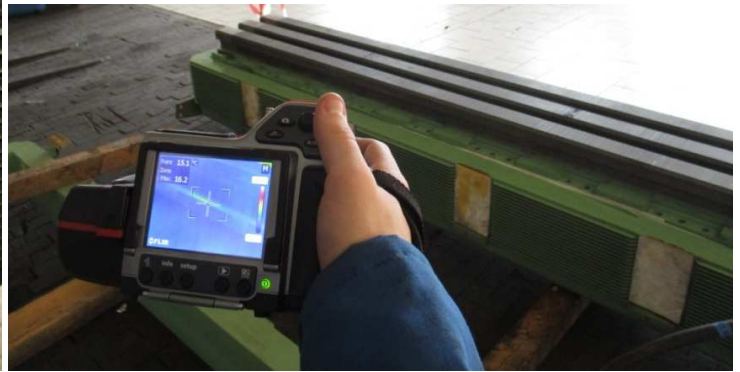
Pole 2 with interturn fault
