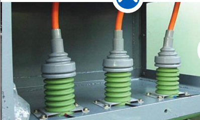
Epoxy Mica Capacitors Installed In Motor Termination Enclosure
