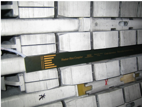
Fig 2: An SSC antenna in the process of being installed on a large generator. A stator wedge is inserted over the antenna.
