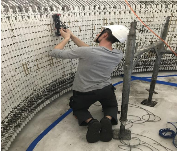
Fig. 8: Scanning of stator core with search coil
