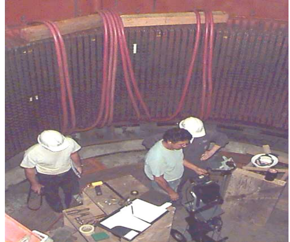
Fig. 10: Rated flux testing with power frequency
