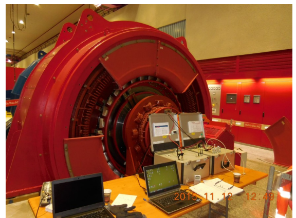
Off-line testing of a stator winding
