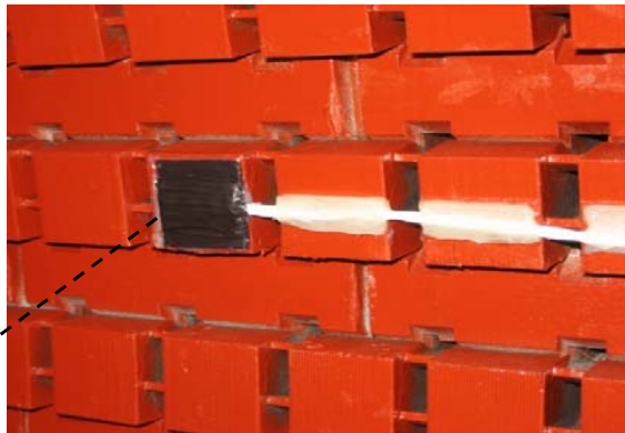
Installation of RFM sensor on air-gap side of stator core
