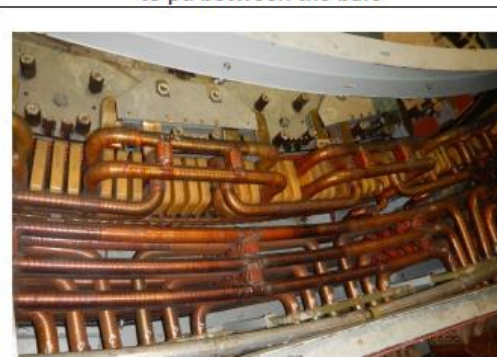
P06: Sections of circuit ring bus discolored – Neutral Side
