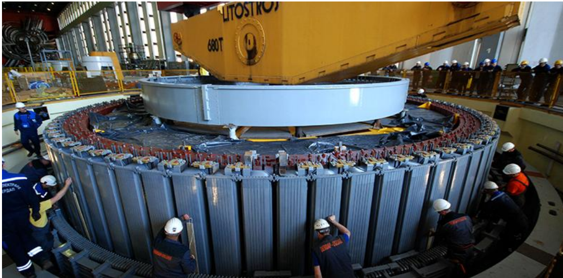
Pict. No. 7 – Positioning of rotor into stator frame with mutual distance of 19mm
