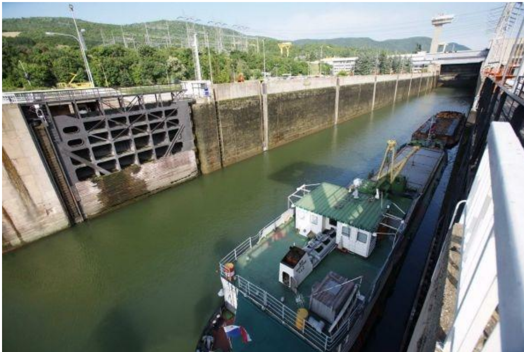
Pict. No1 - Navigation lock for vessels trafficking. With a length of 310 meters and a width of 34 meters, this navigation lock is one of the largest in the world.
