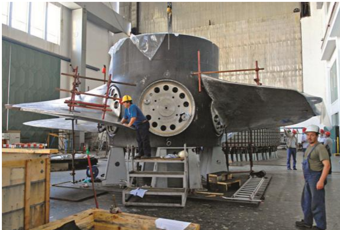
Pict. No. 4 - Only one blade of a steel turbine is heavy at 16.5 tons
