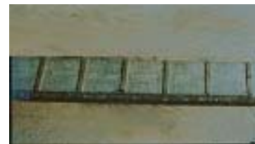
Fig. 1 Photo of a stator bar where the ground insulation was abraded since the bar was loose in the slot.
