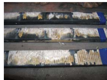
Fig. 2 Stator bar where the slot conductive coating degraded, as a result of poor manufacturing.
