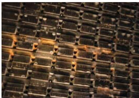
Fig. 3. Wedges destroyed by slot PD.
