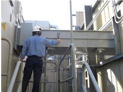
Photo 16. Checking a bus for radiated EMI.
