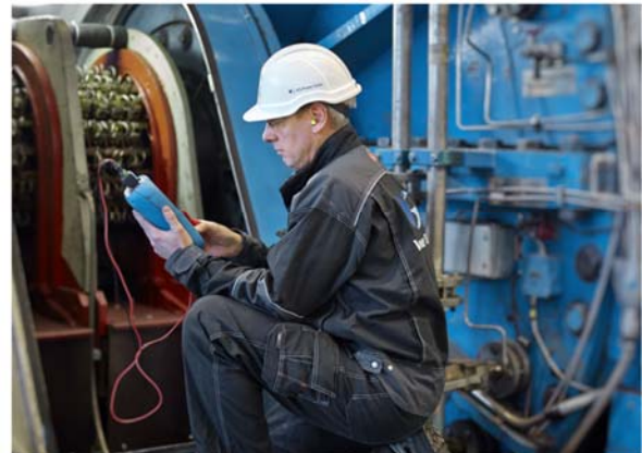
Figure 4 Visual inspection with the trained eye and electrical testing is important parts of the Major Overhaul
