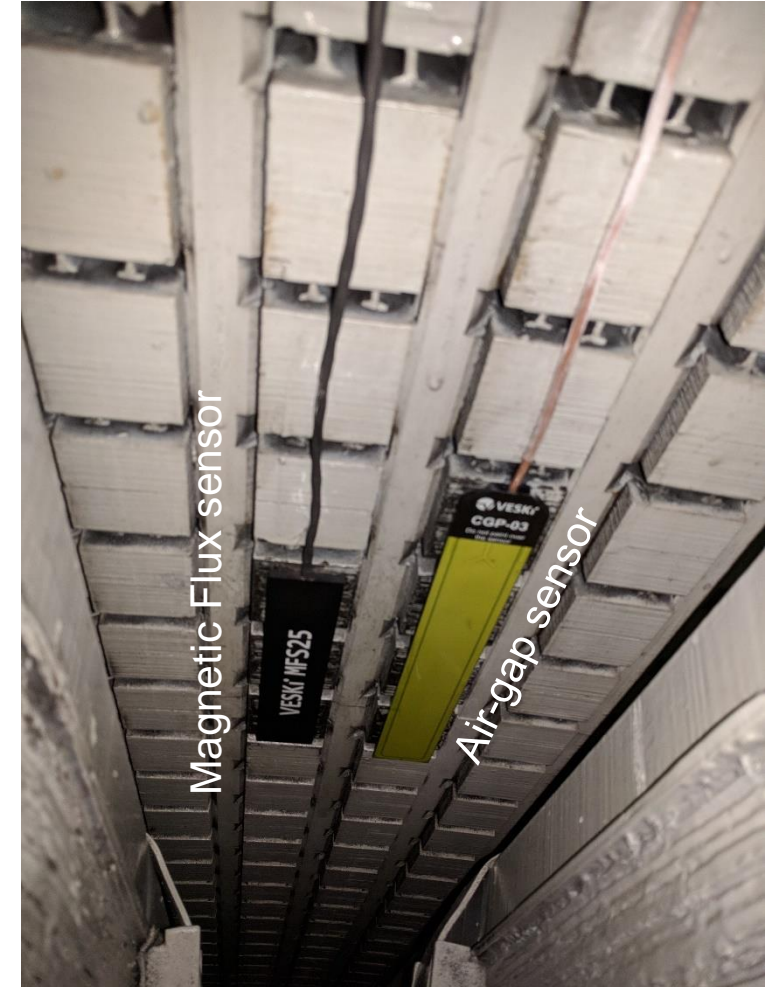
Air-gap and Magnetic Flux sensors
