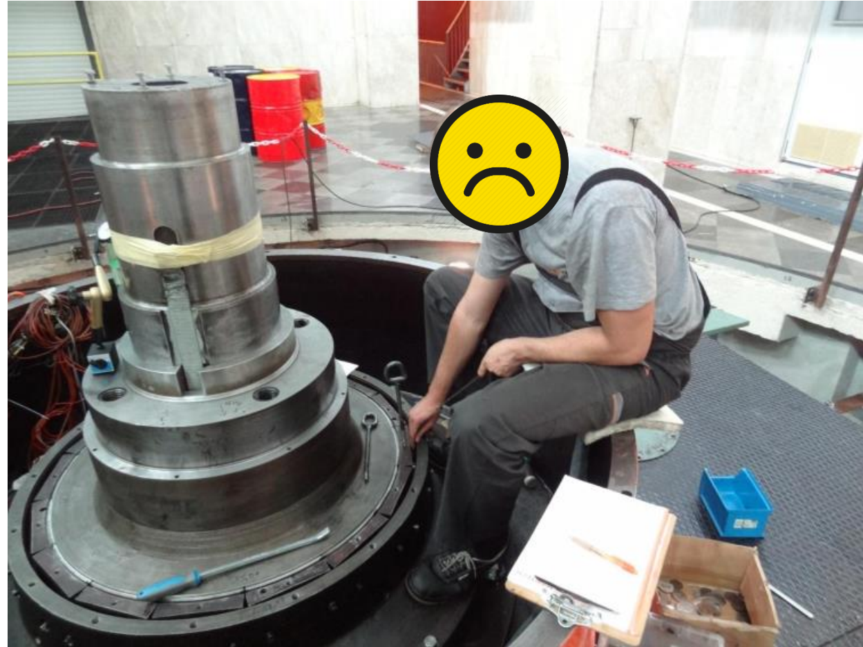
UGB clearance setup during the overhaul
