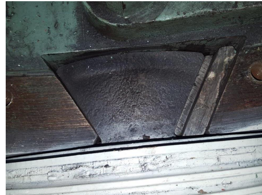
Dovetail connection pole to rim
