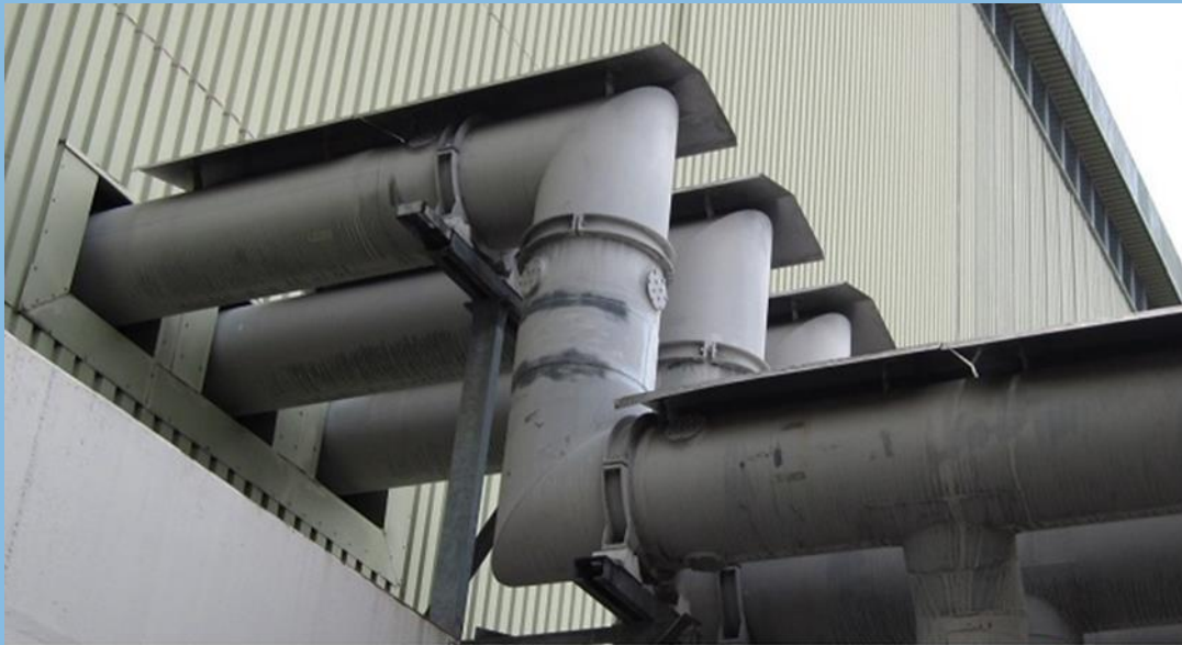
Here the main bus is fitted with a roof for weather protection.
