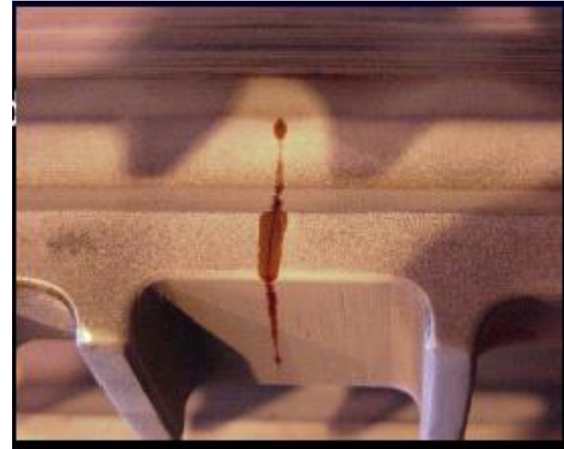
Dye Penetrant of rotor dovetail shows crack
