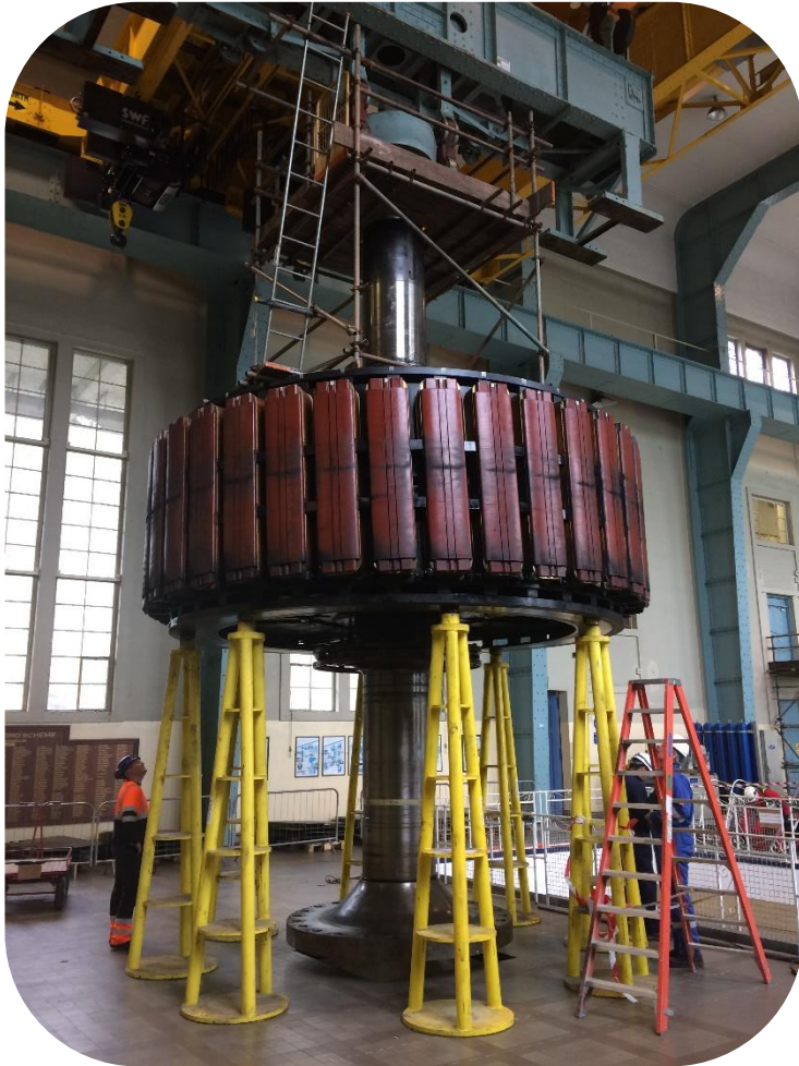
Extracted Rotor
