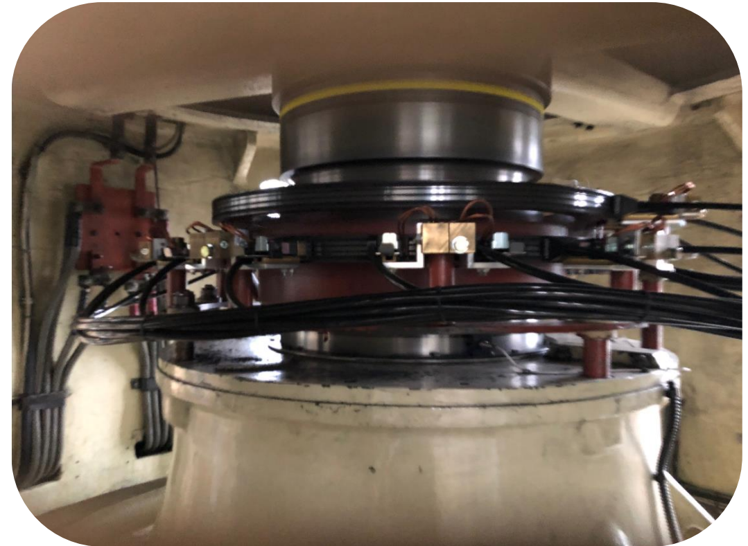
Installation of MERSEN DustCollector Brush Holders
