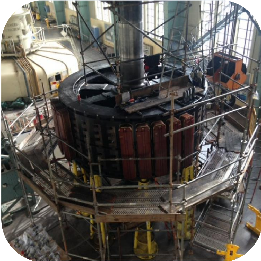
Rotor Poles Disassembly – 36 Poles
