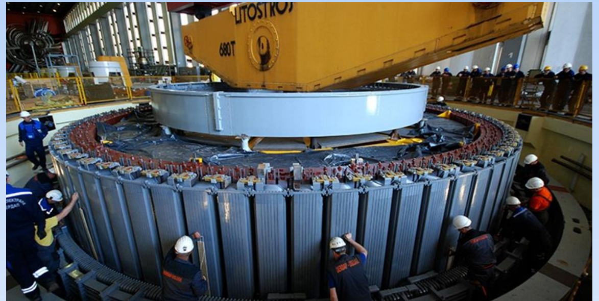
Positioning of rotor into a stator frame with mutual distance of 19mm
