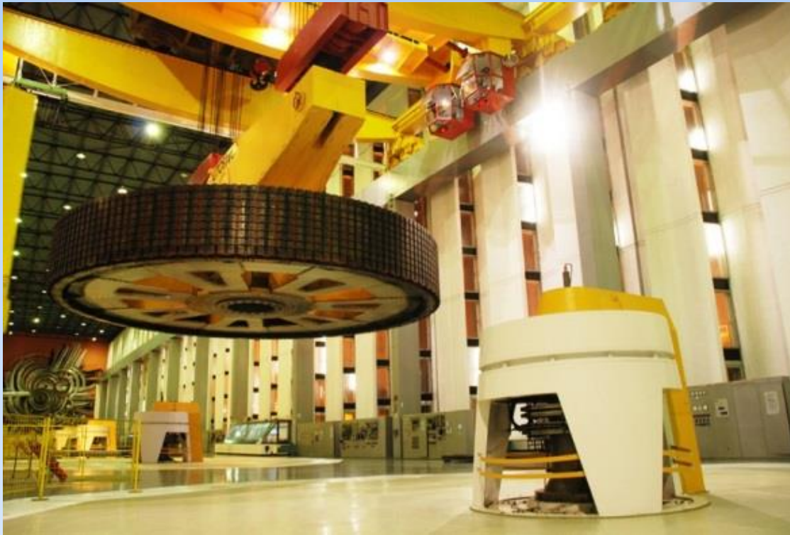
Positioning of stator (G=610t)
