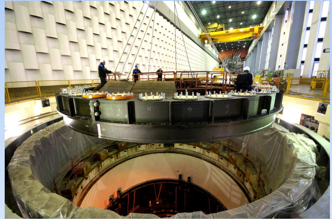
Positioning of rotor
