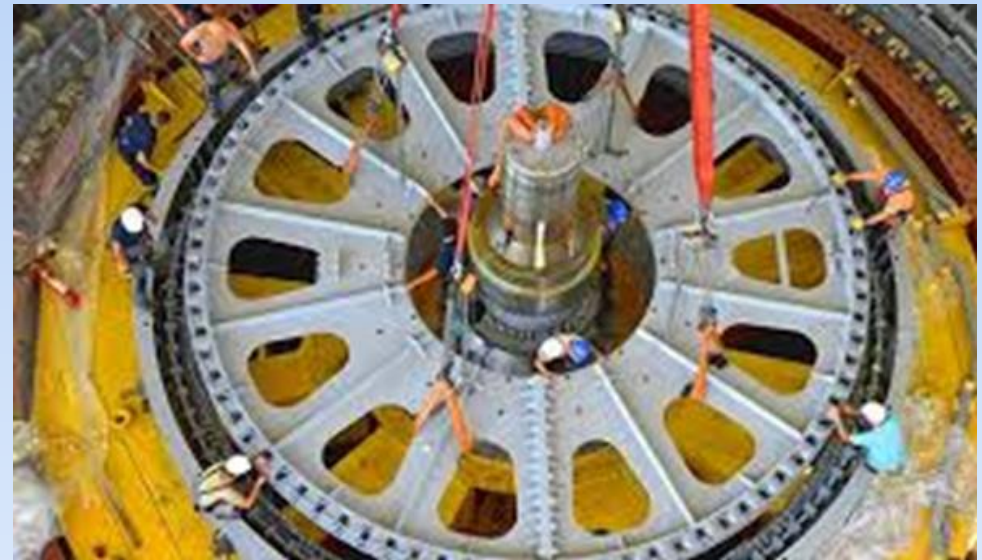
Auxiliary generator erection works
