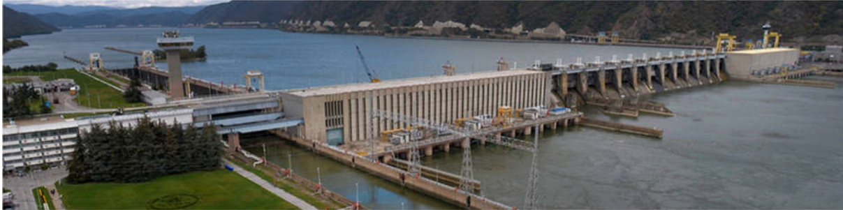
HPP Iron gate 1
