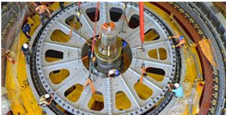
Assembling of new generator
