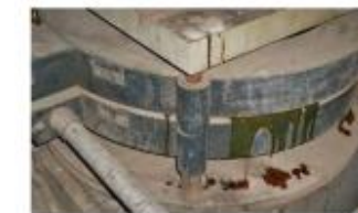
Images from 30020246 showing typical location of generator CTs, type of construction and common heat damage failure mode.
