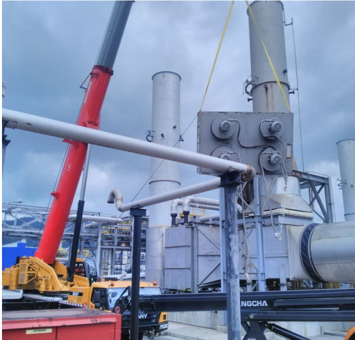
Partial disassembly of the heat exchanger
